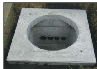
⑩上部部材据付-(2)
