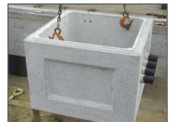
①下部部材据付-(1)
