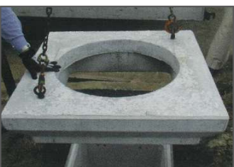
⑨上部部材据付-(1)
